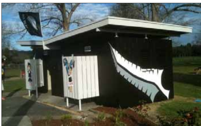
THE RENOVATED KARA PARK TOILETS, PIOPIO
