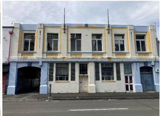
Deteriorating building. Lowe St
